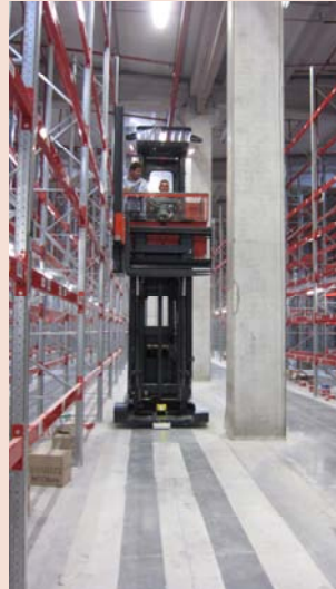
Completed VNA Wheel Track Grinding
