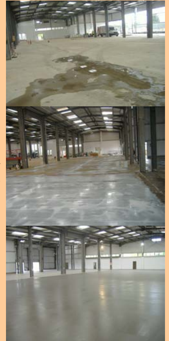
Recent Fastfloor IT project: Laundry Floor Gets Cleaned Up
