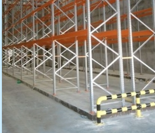
New slab constructed on top of existing floor with racking installed
