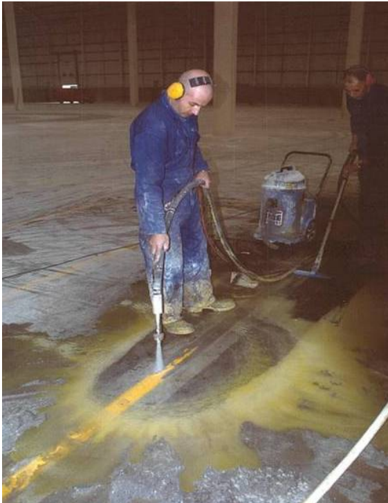
(Soda Jet demarcation line marking removal in progress)
