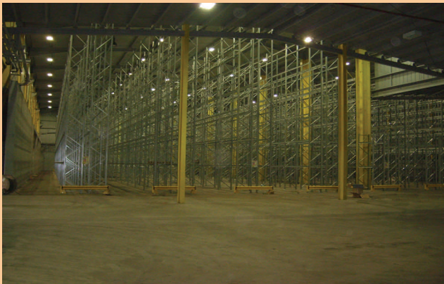
Baxi Warehouse - Floor upgrade completed.
