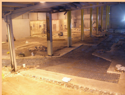
Baxi Warehouse - surface preparation
