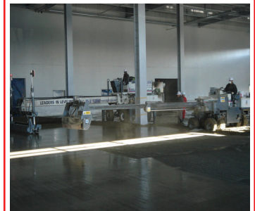
Laser screed and topping spreader in action
