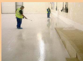
Pump Applied Cementitious Floor Screed
