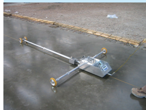
Floor Flatness Testing with FACE Digital Profilegraph
