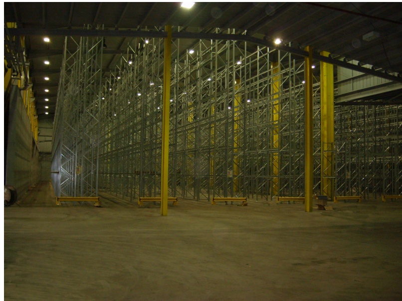
Floor upgrade completed
