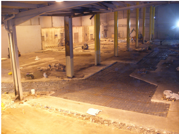
Baxi warehouse - surface preparation
